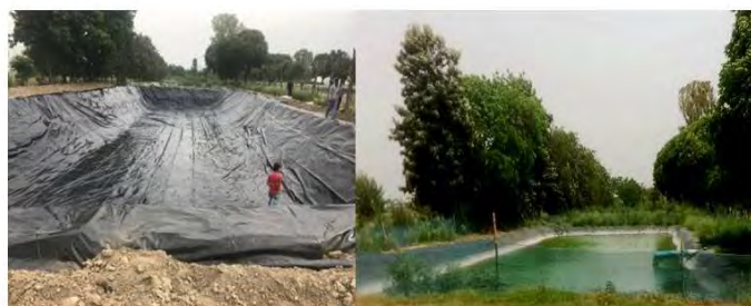
Poly-lined Pond – Seepage Loss Reduction
