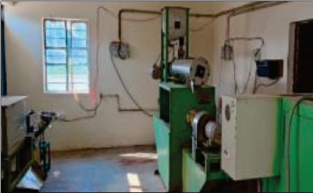
Renovation of Feed Mill at Instructional cum Research Farm, COF
