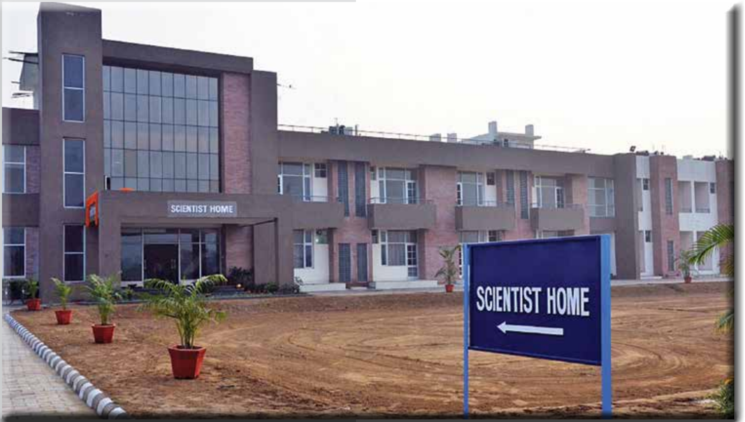
Newly constructed Scientist Home
